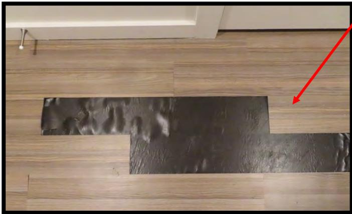
This is a black vinyl foam underlayment where the adhesive just disappeared. The bubbles are from moisture in the slab which then buckled the LVP.
